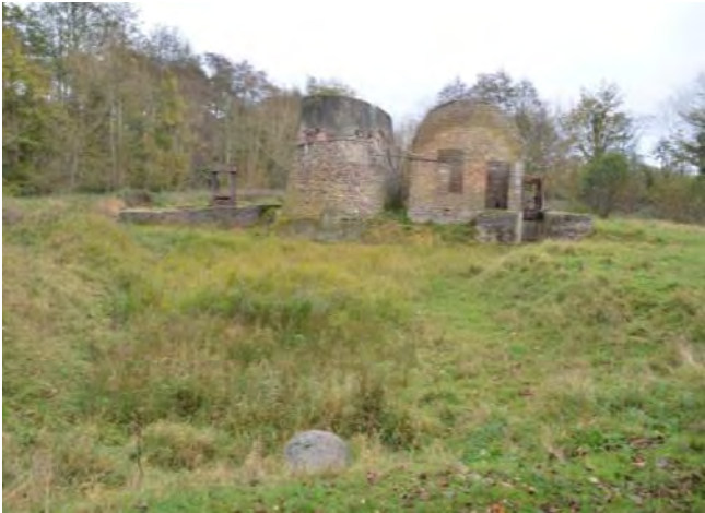
One of the many surviving collection of buildings and structures on the site
