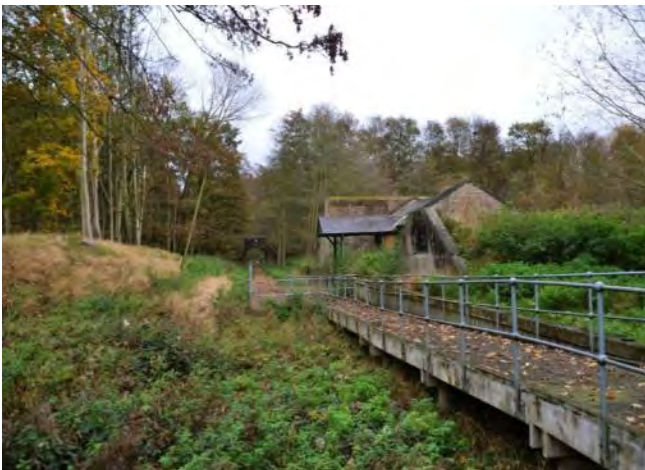
One of the water channels used to transport materials around the site
