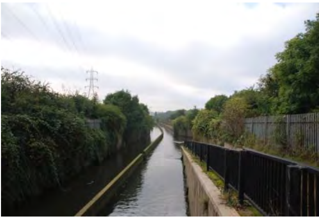
Channelled view along one of the flood relief channels.
