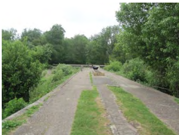
View towards the central well-head of the Middlesex Filter Beds.
