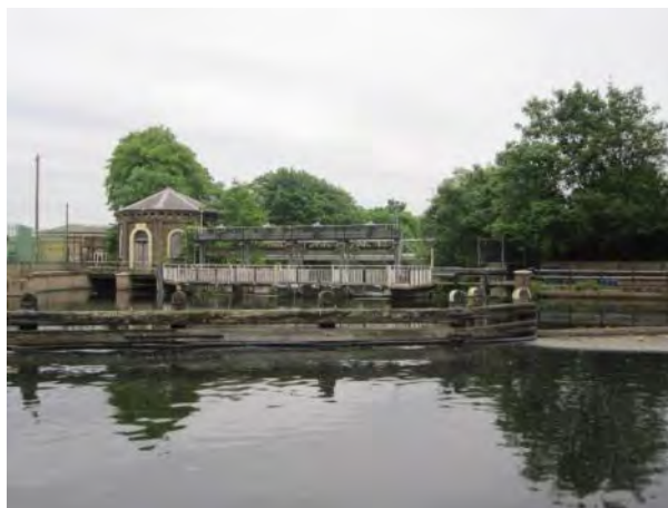
Across the Lee Navigation to the turbine house adjacent to the weir that divides the river in two, marking the beginning of the Hackney Cut of the Lee Navigation (built in the 1790s).
