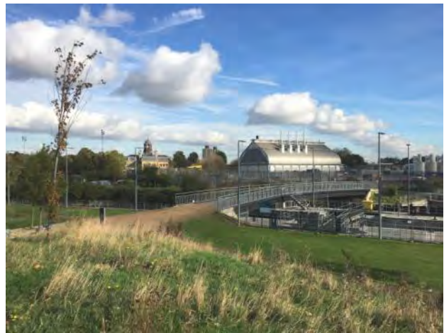
Abbey Mills Pumping Station with its distinctive domed roof, within an industrial context.
