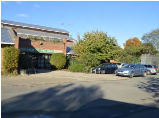
View of the sports centre building.
