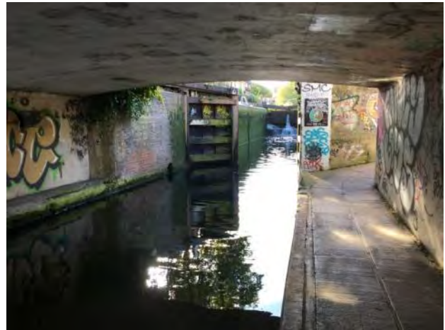
Low bridges over the Hertford Union Canal create confined spaces along the tow path.
