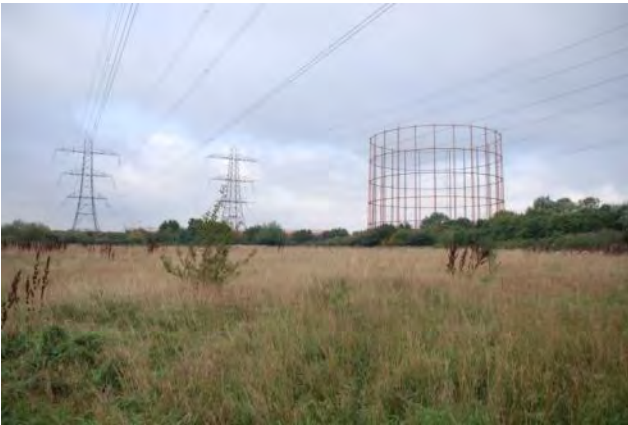
The overhead power lines and gas holder form prominent features on the skyline across the north of the area.
