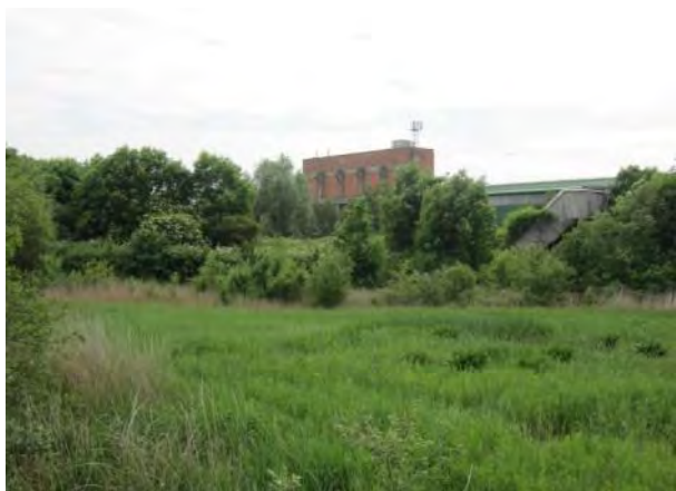
View from within the Middlesex Filter Beds to the National Grid transformer station visible above the tree line to the southwest
