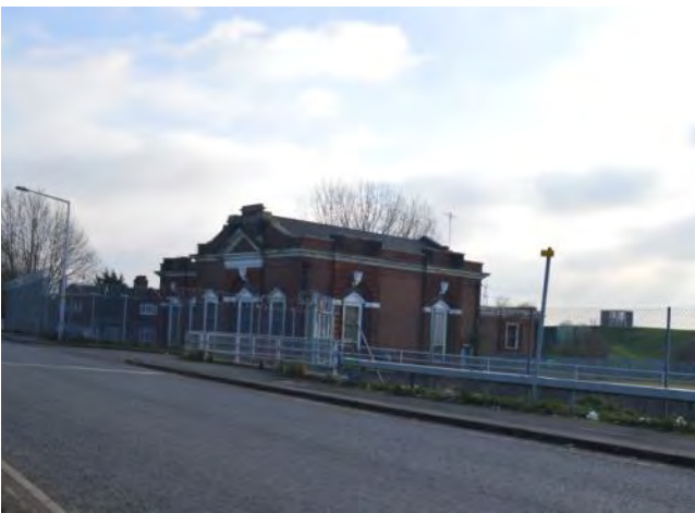
Victorian buildings associated with the original workings of the reservoir (located in the northwest of the area) with the Lee Flood Relief Channel in the foreground and development within Walthamstow visible above the embankment.
