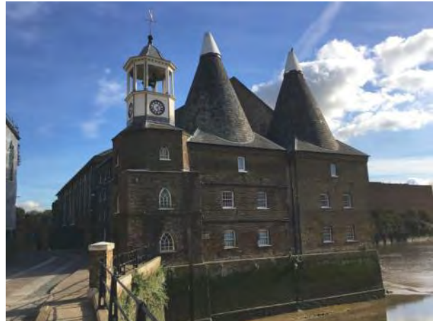
The clock tower and drying kilns (Grade II listed) form distinct local landmarks from the river.
