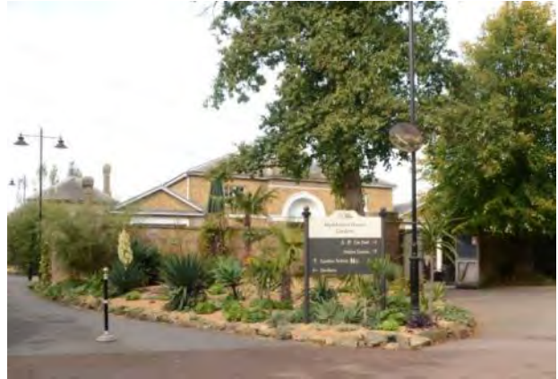
The visitor centre, converted from a Grade II listed stable block
