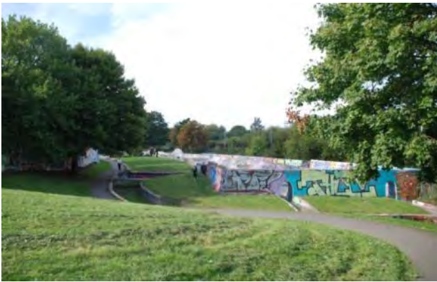
The graffiti walls in the north of the park - the walls and structures of the Victorian Sewage Works still evident
