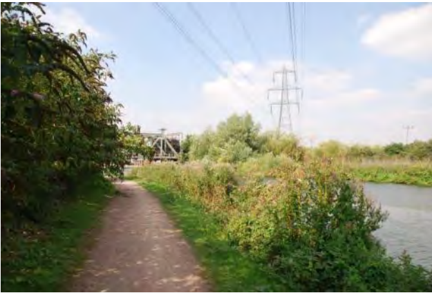
A well-used network of recreational routes, such as NCN Route 1. Pylon lines cross the valley converging at Rye House Power Station and are visually prominent in certain areas.
